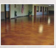
After the final look and color are achieved, L&M Industries, LLC highly recommends the use of a clear concrete sealer. A solvent or water based clear sealer is acceptable, but where permitted, the solvent based sealer proves more durable. The sealer can be applied as soon as the surface has dried. Blot with a white cloth to check. Then follow the manufacturer's guidelines for the application of the clear sealer.
